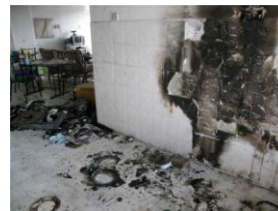
Overloading electrical appliances on a socket could have caused a short circuit in kitchen
