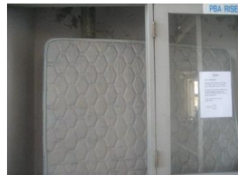
Discarded mattress in the PBA riser
