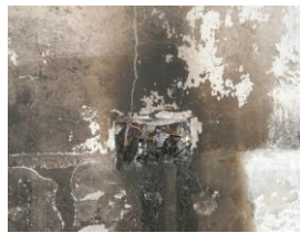
Overloading electrical appliances on a socket could have caused a short circuit in kitchen
