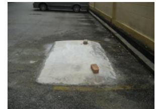
Car park raised up with concrete pad to avoid flood
